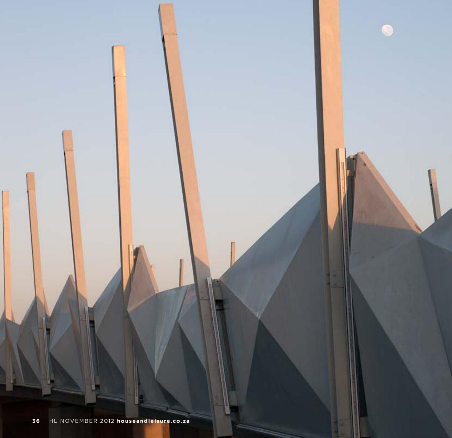
The steel facade of the Nellmapius Bridge on the N1 forms a gateway between Midrand and Centurion. It was inspired by origami and developed using fractal geometry.
